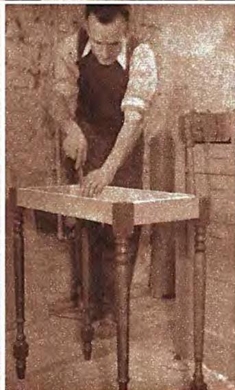
Right: Screwing the arm in place. This holds the rear top panel vertically rigid.
