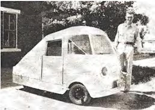
This car attracts a lot of attention wherever Gaylard Train, of Hardy, Neb., drives it. It is a three-wheeled job of his own design and construction. It uses a Model T frame which was shortened and narrowed at the rear end. It is powered by a Harley 74 and has a Harley three-speed transmission. Top speed is about 45 m.p.h. A \$3.00 Workbench check is going out to Gaylard for this snapshot.
